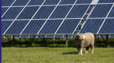
Our panels are ground mounted, installed using pile driven technology which limits the impact on the land. They're installed 80–90cm off the ground at the base with a total height of no more than 3m. Raising the panels off the ground allows sheep or other small flocks to be grazed underneath them. As well as benefitting local ecosystems, conservation grazing helps to control the height of the undergrowth surrounding the panels, meaning less machinery is needed for maintenance.
